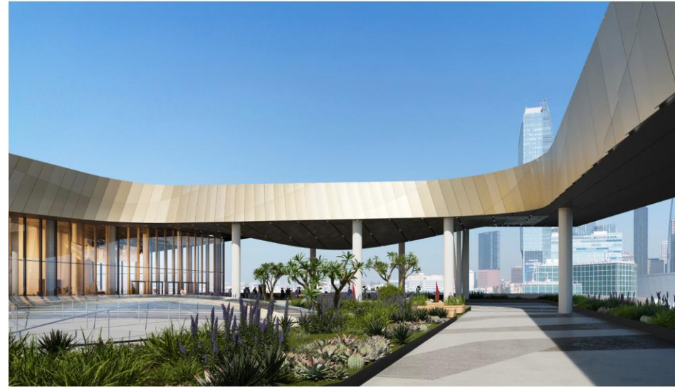
New roof terrace looking north
